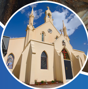
Saint Francis Xavier Cathedral 36 Harbour Street Wollongong
